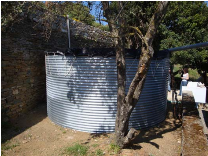
Figure 1. Aluminum water tank at the primary school of Skalados (Tinos) during its installation.
