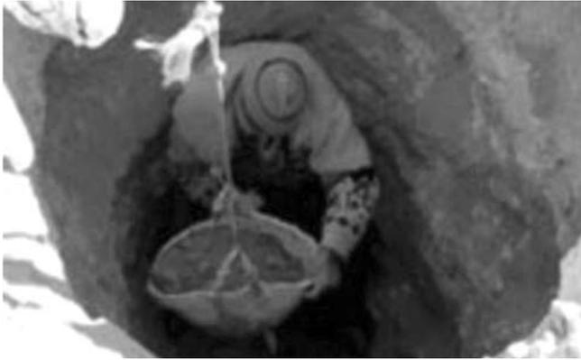
Curetting of a vertical shaft in a foggara
